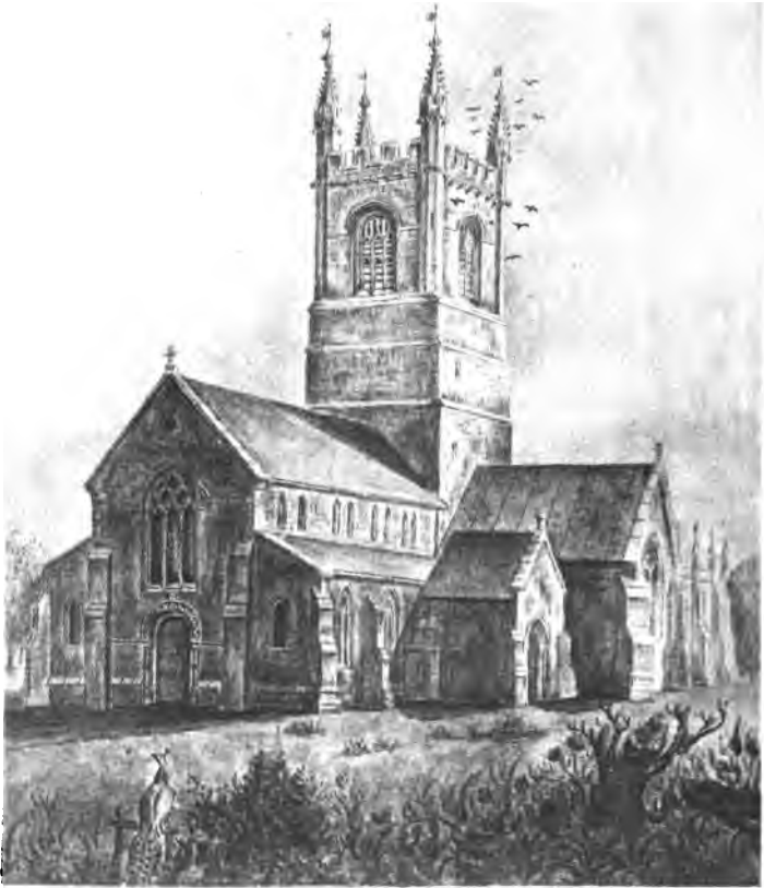
LAMBOURNE CHURCH, WEST VIEW.
